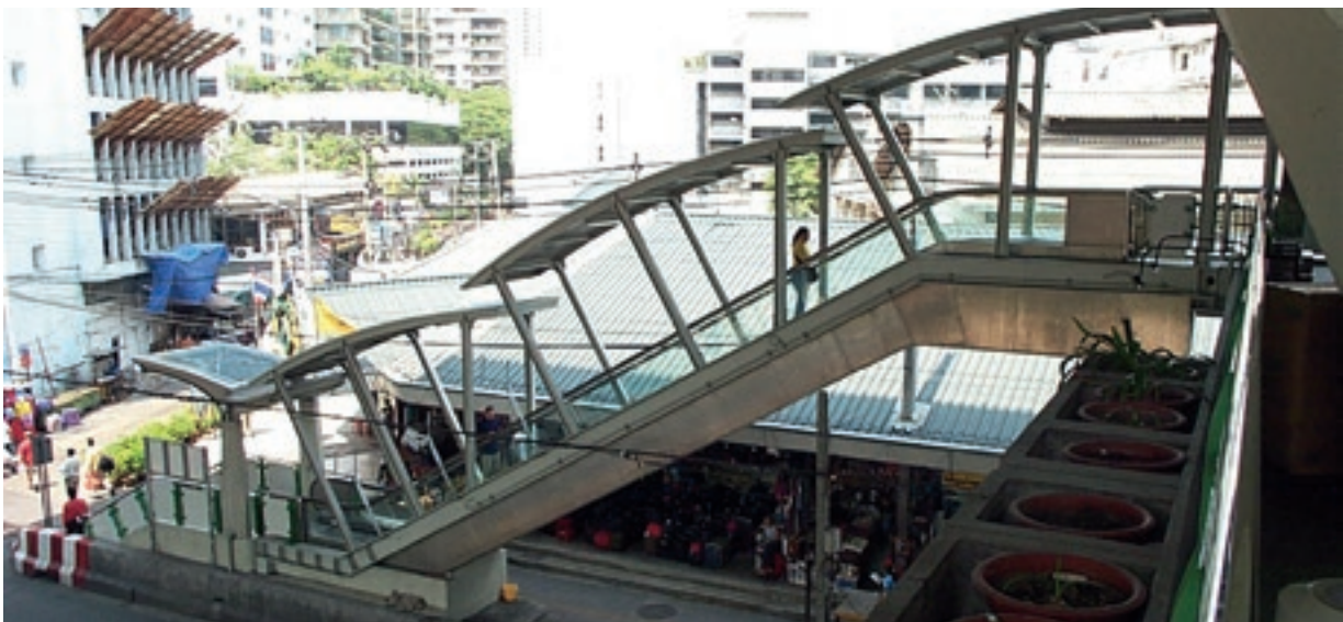
Figure 4.3 The outdoor escalator should be covered by a roof to improve passenger safety and convenience.
