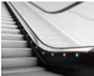
Skirt lighting with spots
