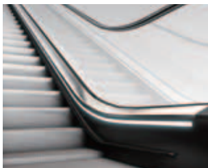
Skirt lighting with light strip
