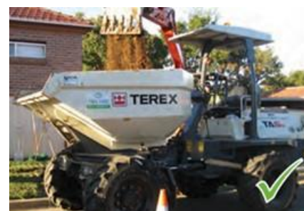
Tipping spoil directly into a truck or skip avoids stockpiling
