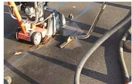
Wet-vac used to collect saw-cutting runoff
