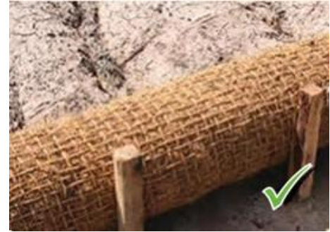
Natural and biodegradable coir logs can be used on unsealed surfaces
