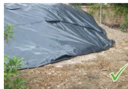
Stockpile covered with plastic to prevent wind and water erosion
