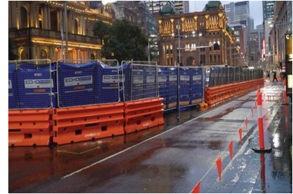
Portable noise screen used to mitigate noise
