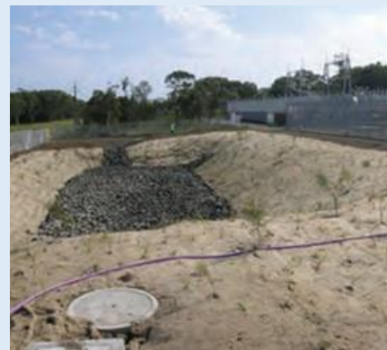
Rehabilitate disturbed areas to prevent erosion
