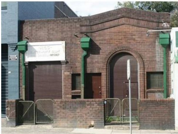
Ausgrid S170 heritage substation. Also, Local heritage
