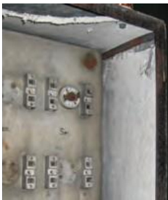
Millboard lining inside the fuse box
