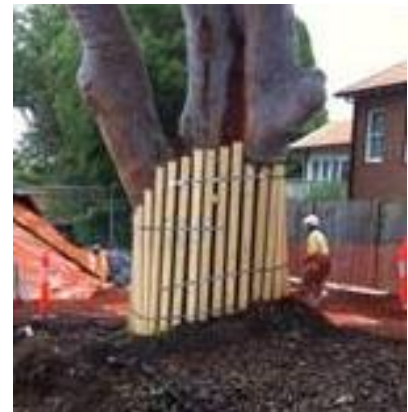
Strap boards and padding to the trunk to prevent damage
