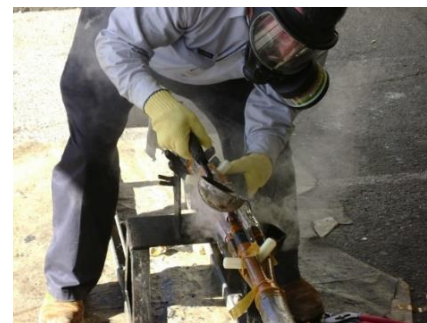
Lead wiping a cable joint
