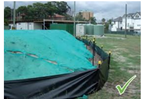
Stockpile covered to prevent dust and sediment fence used to filter runoff
