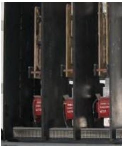
Zelemite board phase barriers
