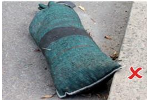
Fill geotextile filter bags to two-thirds capacity so they can be keyed firmly against the kerb
