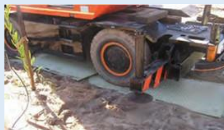
Temporary construction mats help minimise ground disturbance
