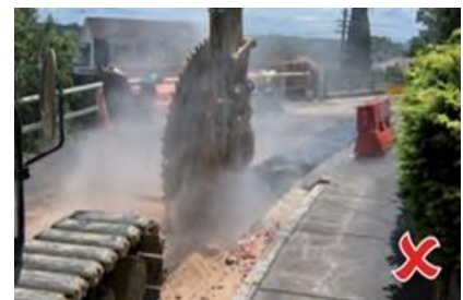
Prevent dust from leaving the worksite
