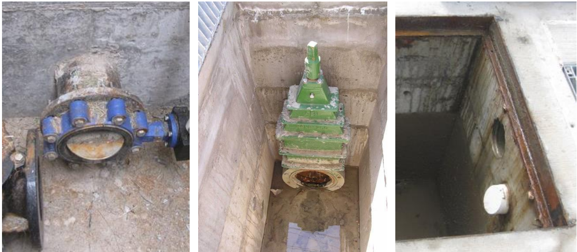
Figure 12: Butterfly, Knife Gate and Reflux Valves (left to right)
