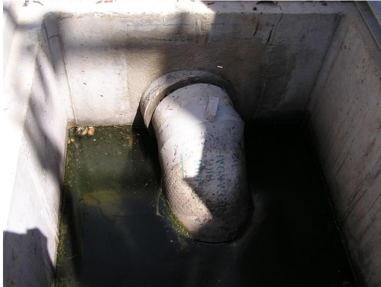
Figure 6: Typical Flame Trap (grate removed for photo)
