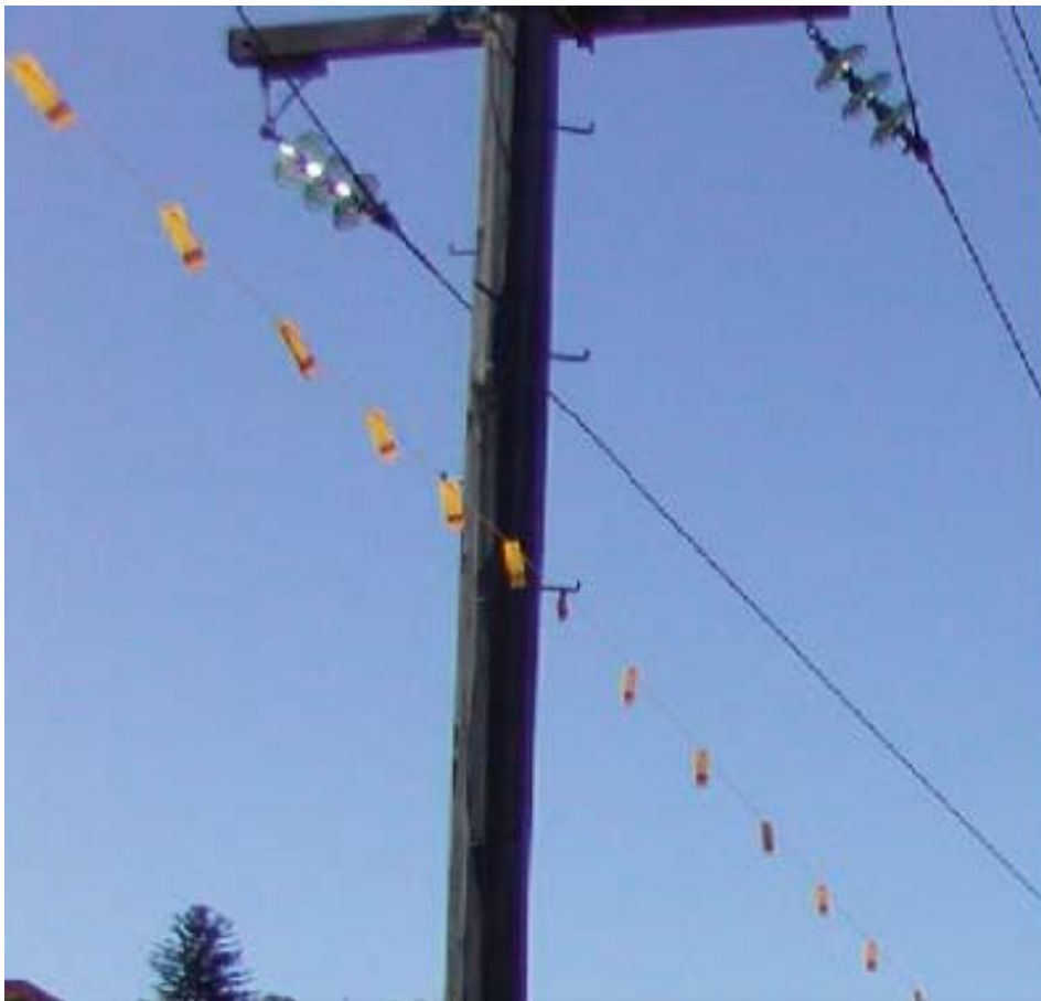
Figure A 3 – Illustration of a visual tape bunting fitted under overhead power lines.
