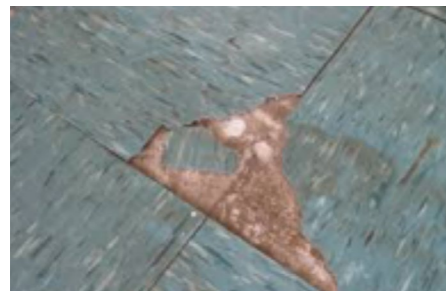
ACM floor tiles
