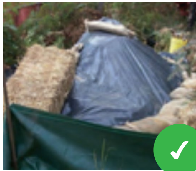
Stockpile ASS/PASS correctly to minimise exposure to air
